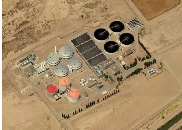
Figure 1: El Paso Bustamante Wastewater Treatment Plant
