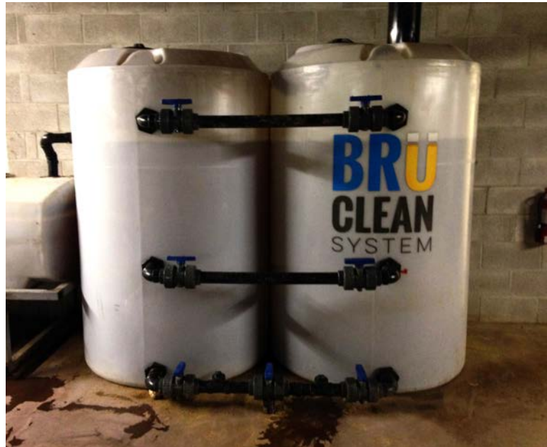
Installed BRÜ CLEAN Pilot Balancing Tanks
